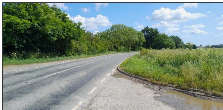
View east along B1200 from site entrance
