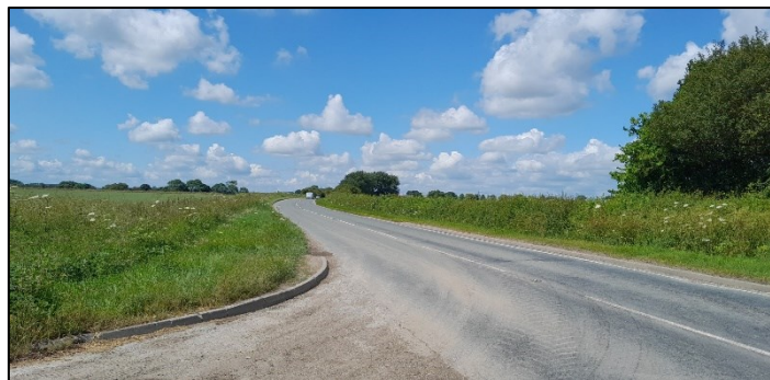
View west along B1200 from site entrance
